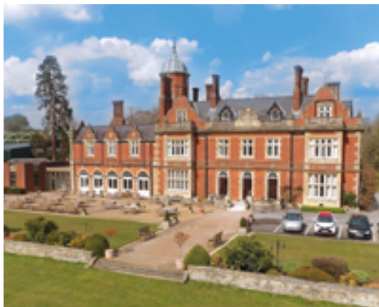
Howbery Park, QE head office location
